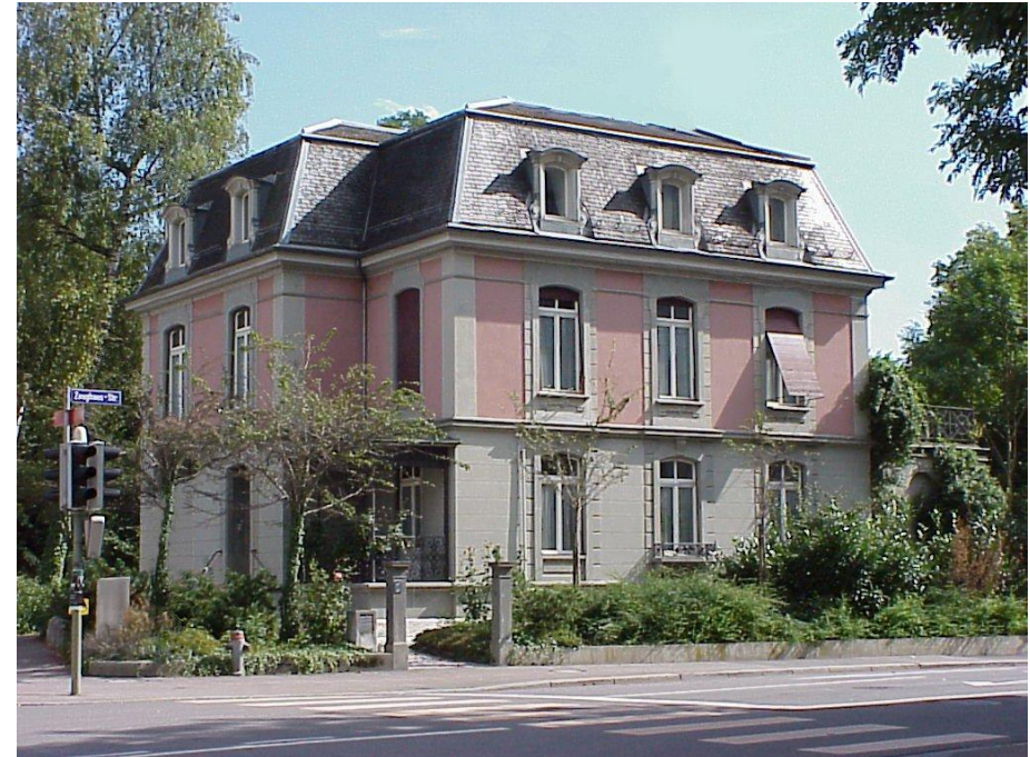
IMS-Building Villa Forrer
